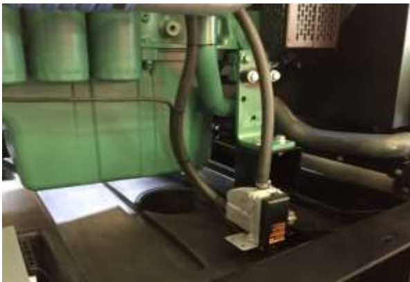
ESTERNAL HEATER (i.e. as general reference)
