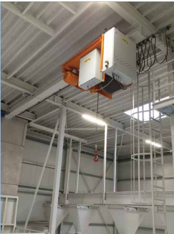
SB-E307 as a mobile rope hoist
