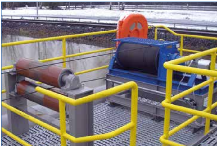
SB-E 304 as a traversing winch for a water treatment plant
